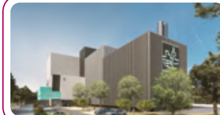
IDEX wins the contract to build a new Energy-from-Waste (EfW) plant in Labeuvrière.
